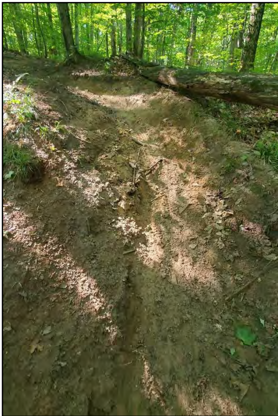
Photo 12. Severe erosion of new trail section built over sand.
