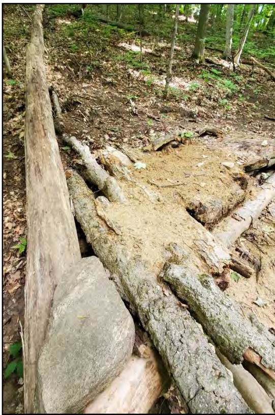
Photo 10. Soil and roots displaced from forest floor to enhance log-over structure.
