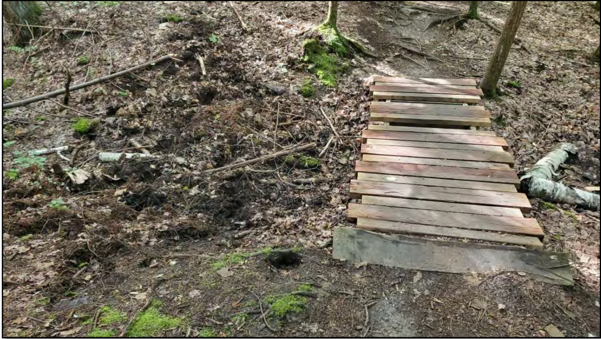
Photo 17. Horses mucking in seepage beside footbridge on single-track trail.
